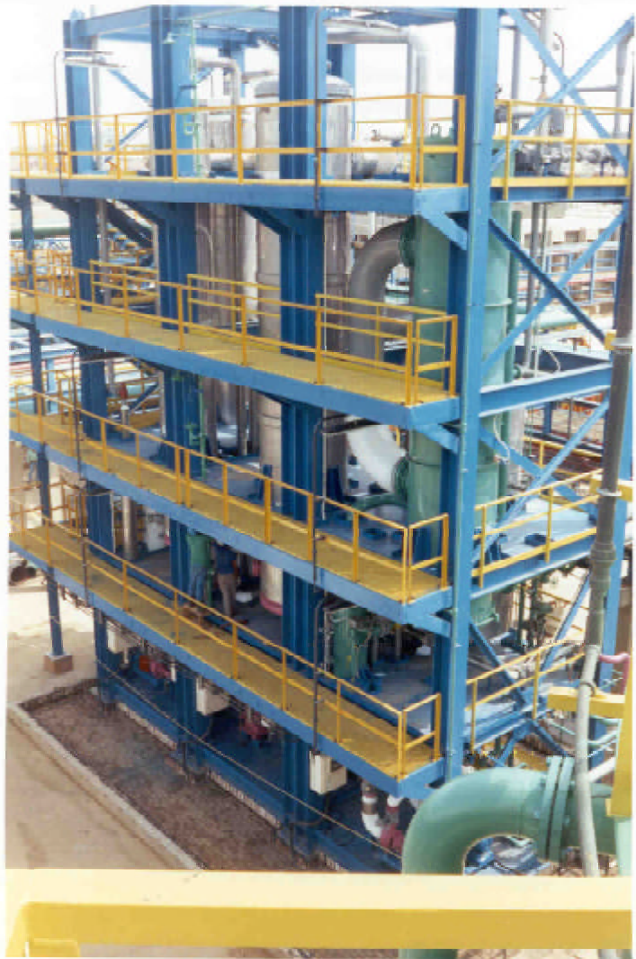
Three-effect 20,000 kg/h caustic soda evaporator installed at a chemical complex in Maracaibo, Venezuela.
